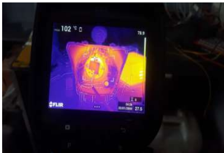
Fig 4 Temp At Source Using Thermal Imaging Camera
